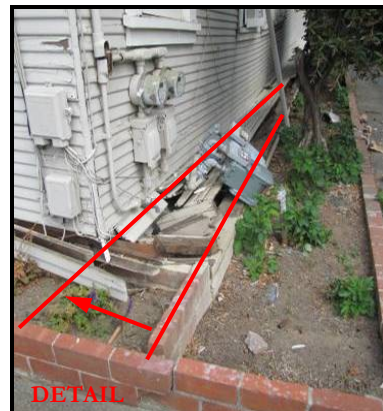
Residential wood-framed structures that predate modern seismic design consideration can shift from their foundations when short wood-framed walls are present surrounding the crawl space below the main floor. These common failures can lead to a fire-following-earthquake hazard from severed natural gas piping and nearby electrical components. Correcting this condition involves installation of plywood sheathing with floor and foundation connections.
