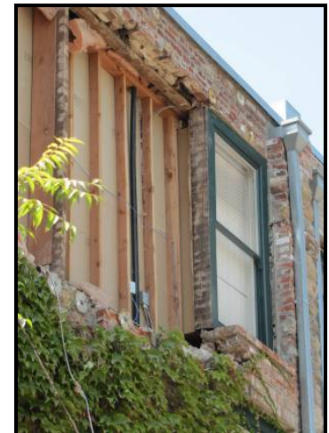
Masonry wall failure in a building retrofitted with wall anchors at roof and floor levels.
