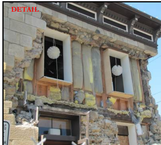
Damaged 1875-vintage stone masonry building in Napa. Note wall anchorage (through bolts with steel plates) in the close-up photo
