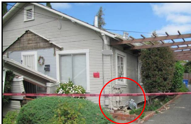
Residential wood-framed structures that predate modern seismic design consideration can shift from their foundations when short wood-framed walls are present surrounding the crawl space below the main floor. These common failures can lead to a fire-following-earthquake hazard from severed natural gas piping and nearby electrical components. Correcting this condition involves installation of plywood sheathing with floor and foundation connections.
