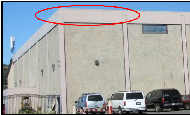
Proactive upgrades of reinforced concrete tilt-up structures can be effective in preventing roof and wall separation. This building in Napa that survived the earthquakes was retrofitted with wall-to-roof thru-bolt connections.
