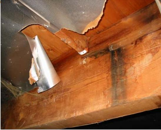
If you can see a white surface at the bottom of the sub-purlin hanger(s), the condensation process is affecting these hangers as well. In more severe cases, the sub-purlin hanger is rusting and is becoming ineffective.
