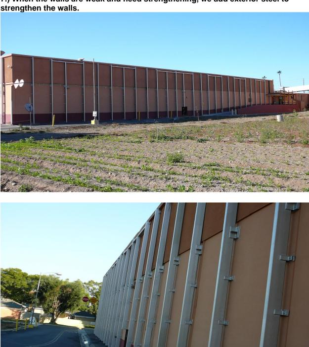
7.) When the walls are weak and need strengthening, we add exterior steel to strengthen the walls.
