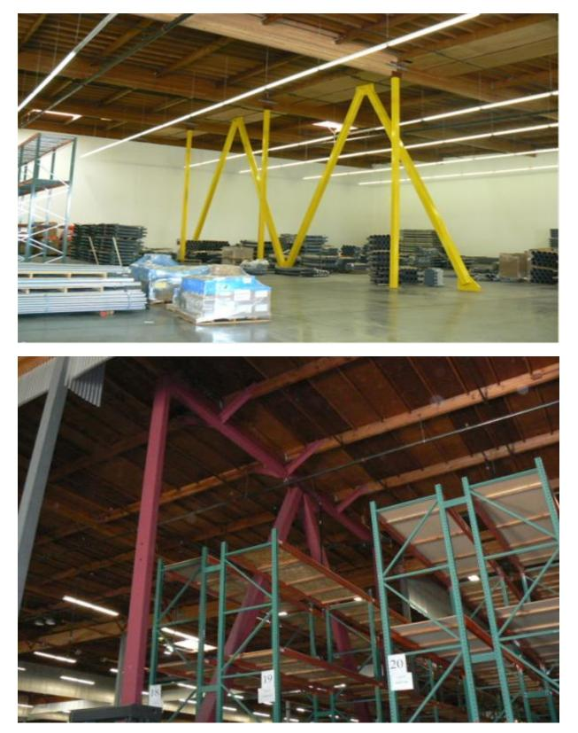
Large brace frame connected to a roof drag line to distribute the forces.
