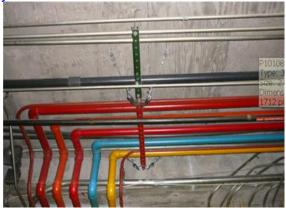
Protecting the operations of a business along with the building by equipment anchoring.
