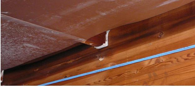
(Notice the white corrosion formed on the sub purlin hanger)
