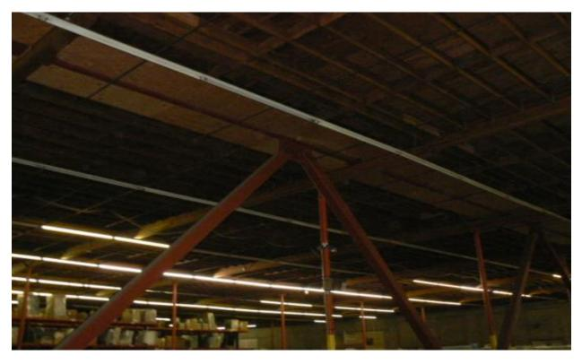
Bottom section of a brace frame in an existing office area.
