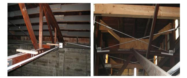
Venting the foil can greatly reduce the chance of Condensation problems continuing or starting. Cutting back the foil approximately 3 inches from the ends lets the cavity breathe.
