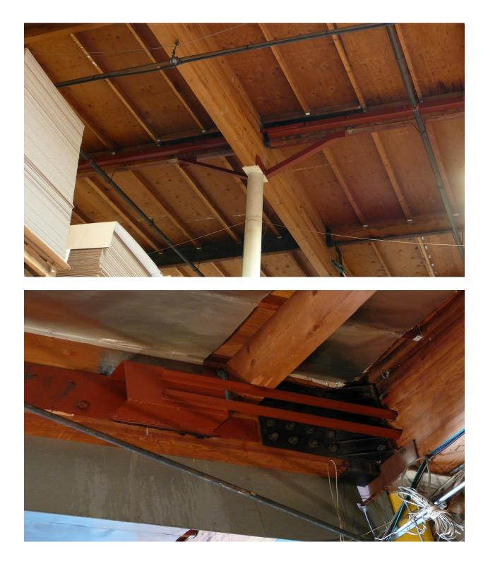
**5. When needed a brace frame or shear wall is added** (This usually needs to be done when the length of a building is three times longer that it's width).
