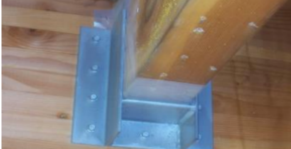
New custom retrofit hanger
