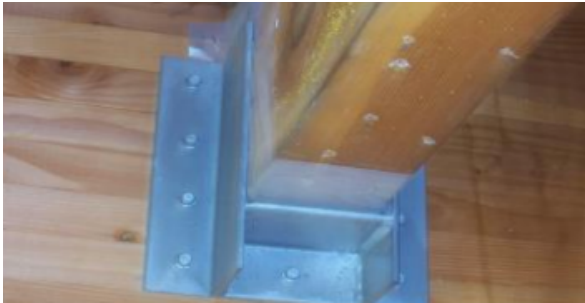
New custom retrofit hanger
