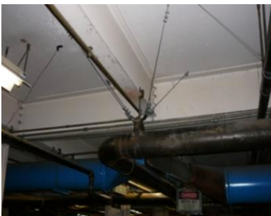
Tube steel frame bolted to concrete floor for secure tank containment.
